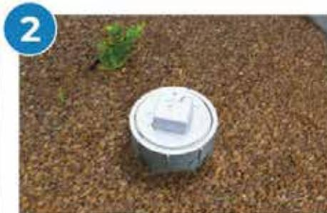
2 For most in-ground pools, use built-in line to drain through sanitary sewer cleanout.
